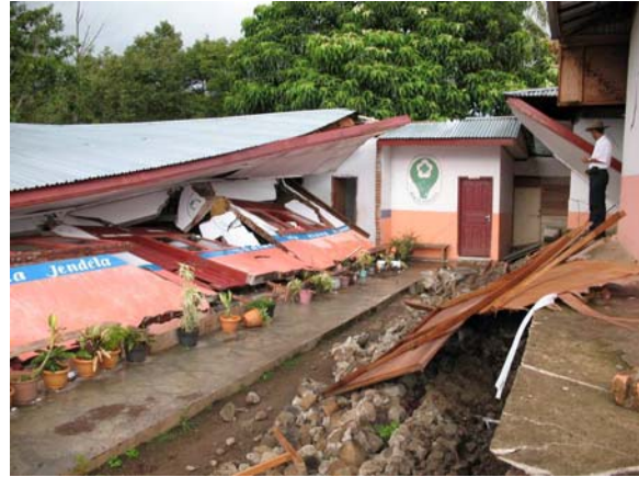
b. Out-of-plane failure of URM wall
