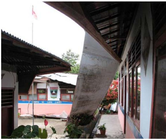
c. Soffit failure
