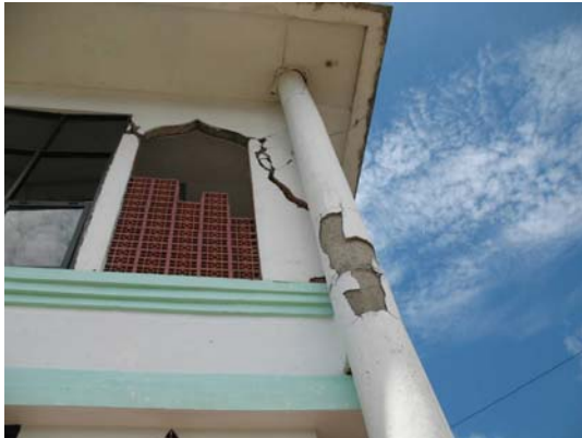
a. Concrete spalling of slender columns
