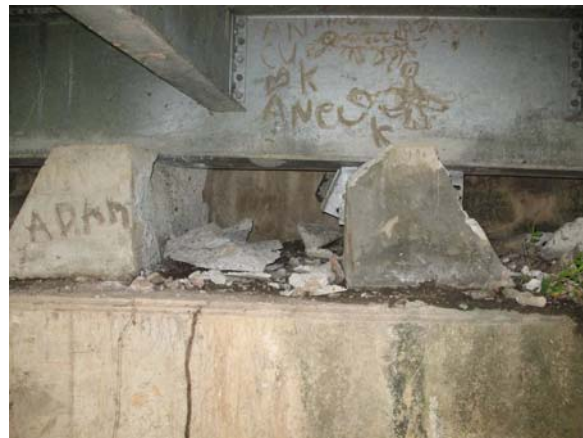
d. Shear key failure
