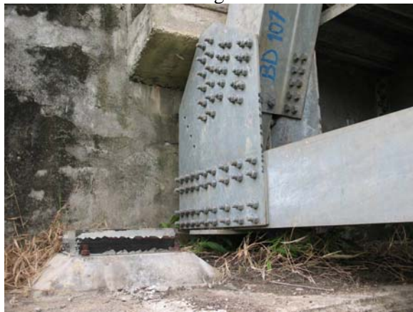
c. Transverse movement off bearing pad
