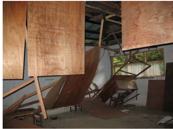
d. Ceiling damage
