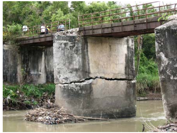
b. Shear failure
