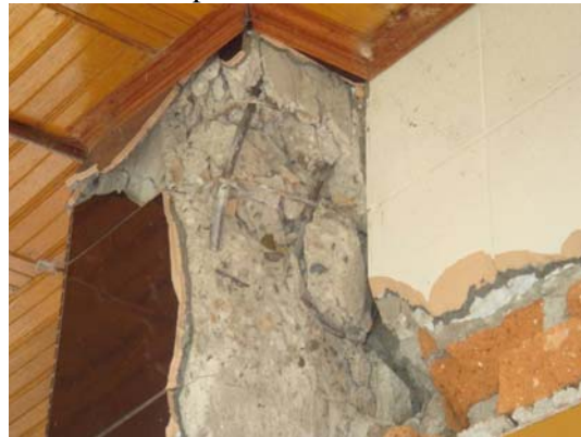
d. Beam-to-column joint failure
