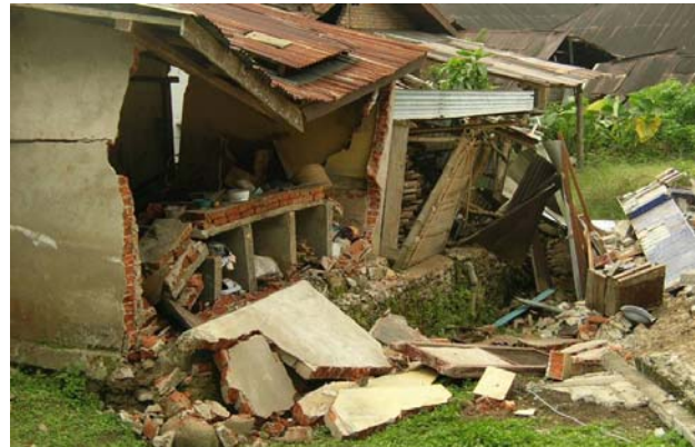
b. Out-of-plane failure of URM wall
