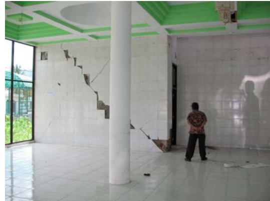
b. URM failure
