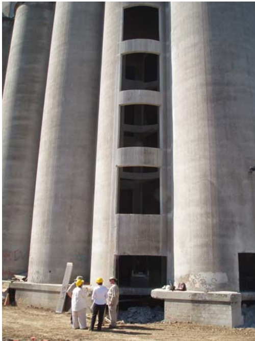
Figure 10. Openings in the Silo
