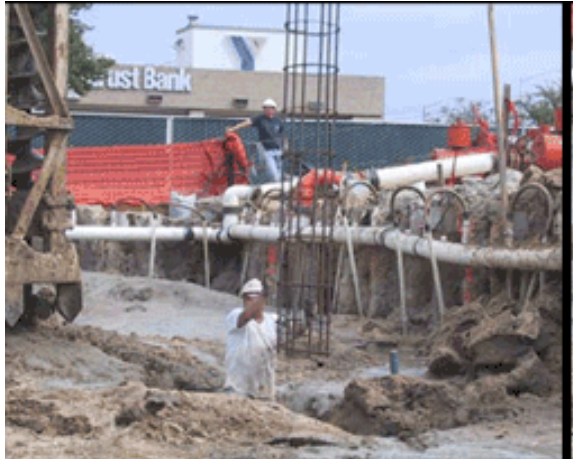
Figure 40. Placement of Reinforcement Cage
