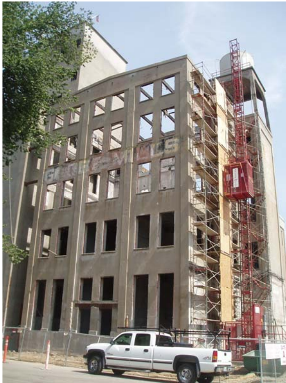
Figure 15. Mill Building Prior to Retrofit (Leaning Left)
