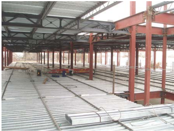
Figure 27. Columns of Truss Moment Frames
