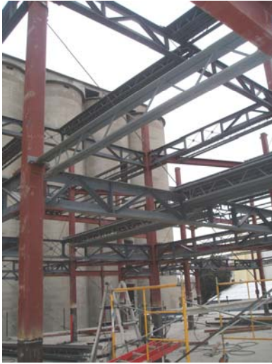
Figure 25. Typical Truss Moment Frames
