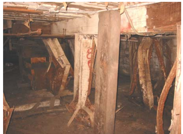
Figure 14. Failure of Existing Columns
