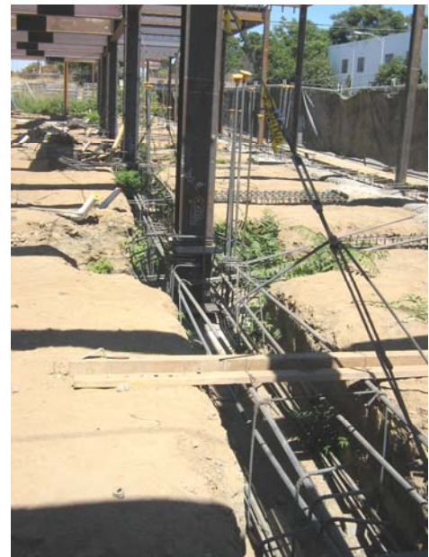
Figure 21. Foundation Construction for Podium
