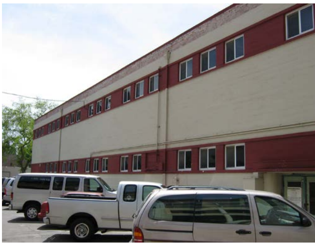
FIGURE 1 PHOTOGRAPH OF THE BUILDING
