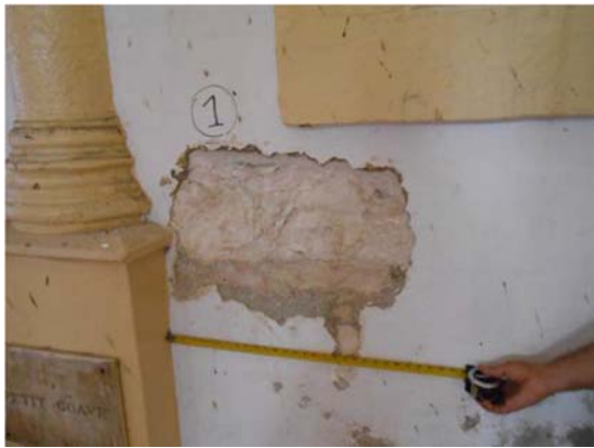
Irregular-shaped stones placed in the mortar
