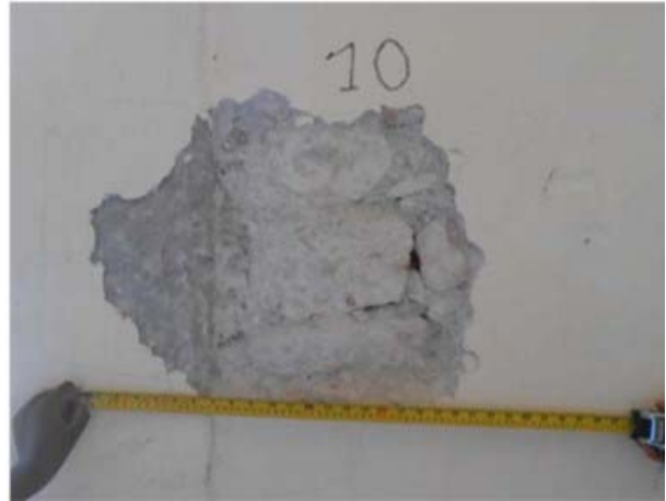
Rectangular-shaped stone and debris in mortar
