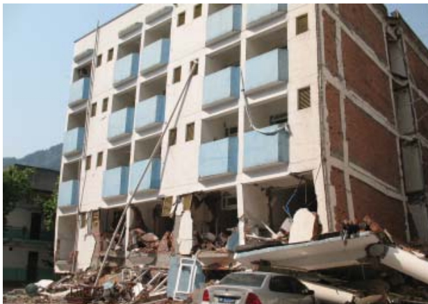
Figure 19. Soft Story Collapse of Hospital Building
