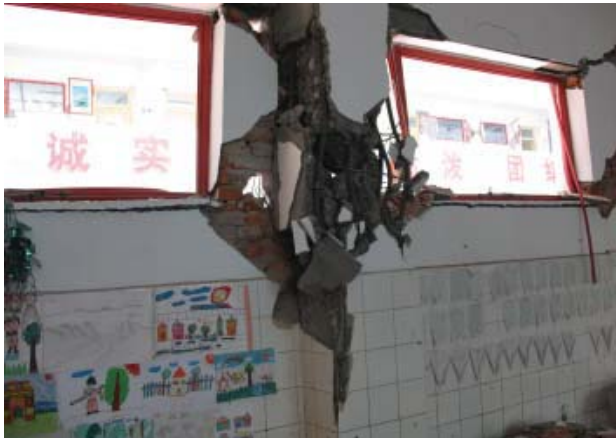
Figure 14. Captive Column Failure
