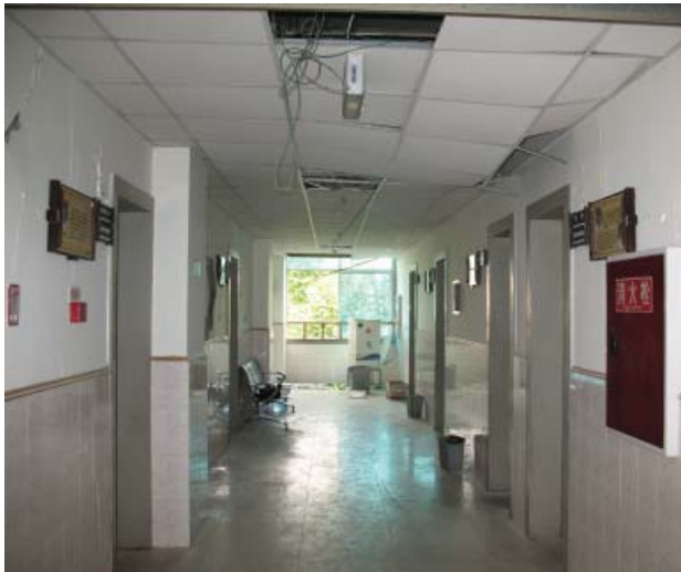
Figure 18. Nonstructural Damage
