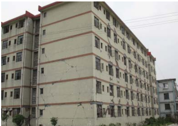
Figure 15. Cracked URM Walls
