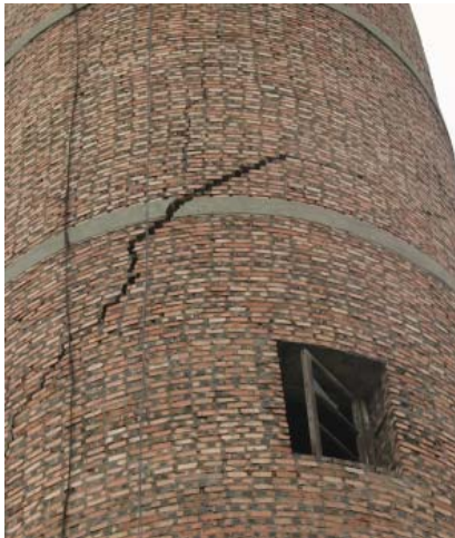
Figure 39. Large Shear Crack in URM Water Tower
