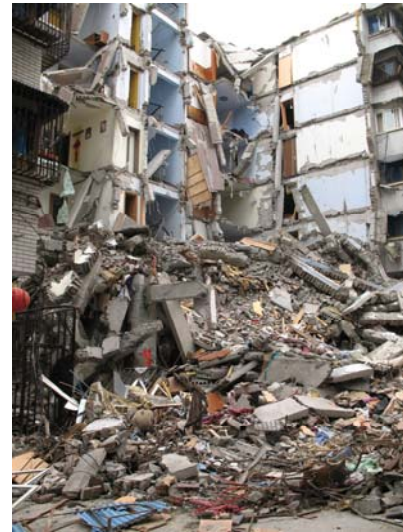
Figure 27. Collapsed Corner of the Building
