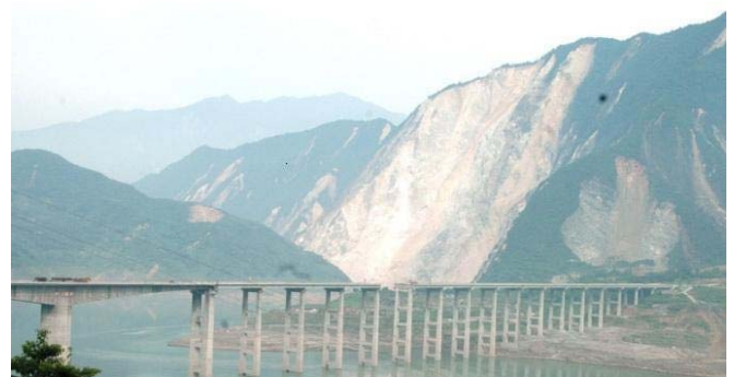
Figure 34. Bridge with Un-Seated Span (NCREE)
