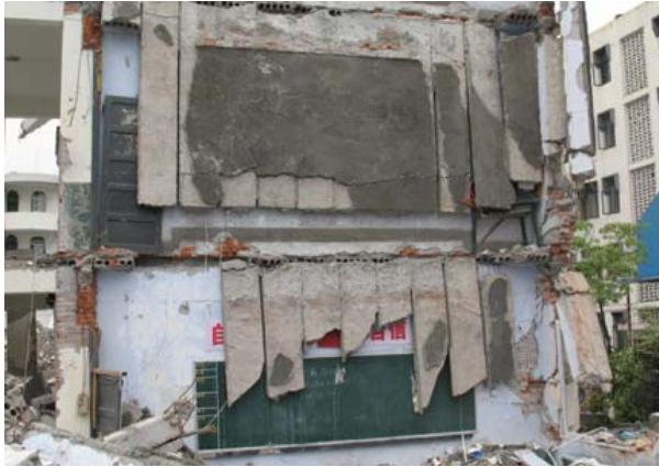
a. Collapsed Floor Planks
