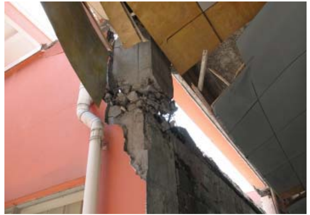
Figure 16. Column Flexural Failure
