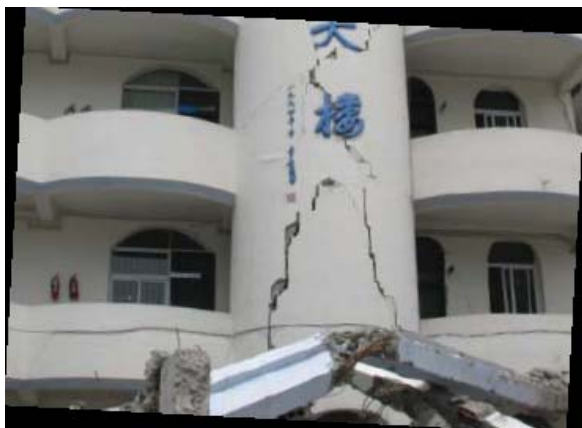
Figure 11. Shear Cracks in Masonry Walls
