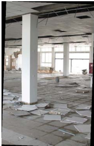
Figure 26. Damaged Suspended Ceiling
