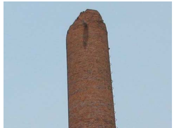
Figure 20. Damaged URM Stack
