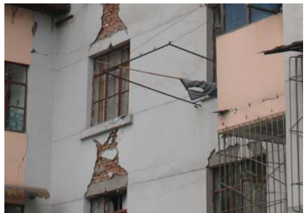
Figure 31. Cracked URM Walls
