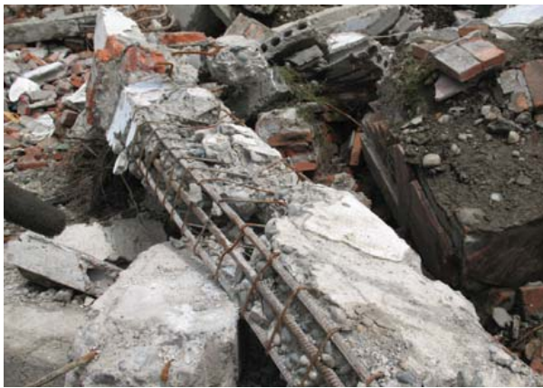
b. Collapse URM Wall and Concrete Beam
