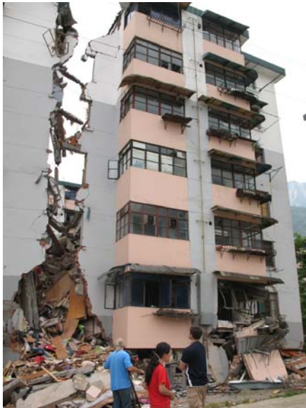
Figure 32. Vertical Split and Displaced Apartment Complex
