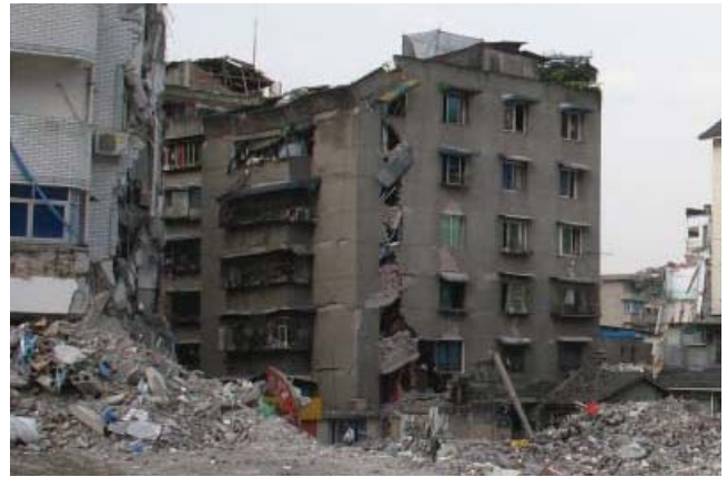
Figure 17. Collapsed Hospital Wing
