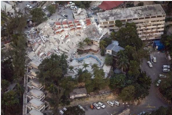
Figure 1 Collapsed UN building (UNDP Global 2010)
