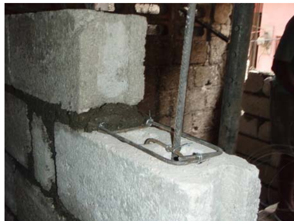
Figure 5. Example of acceptable reconstruction in Haiti
