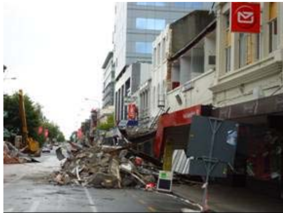
Figure 3 Collapsed masonry buildings in the CBD
