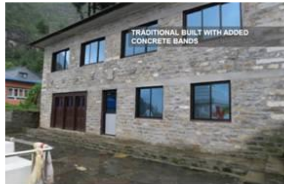
Fig. 8 Building with concrete band
