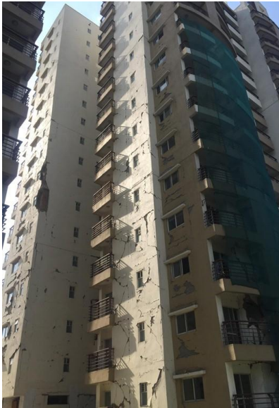
Fig. 11 Exterior cracking, residential tower
