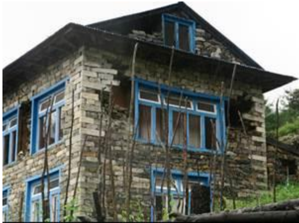
Fig. 9 Out-of-plane failure of bearing wall building
