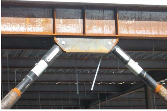
Figure 1. Steel SMF with dampers
