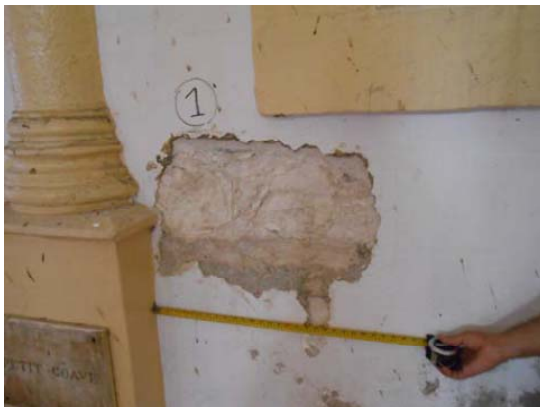
Irregular-shaped stones placed in the mortar
