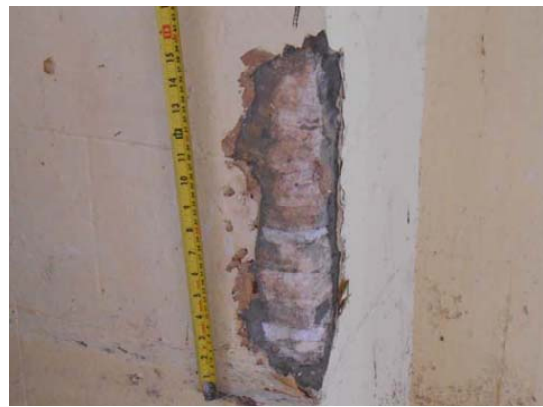
Rectangular-shaped stone and debris embedded in mortar
