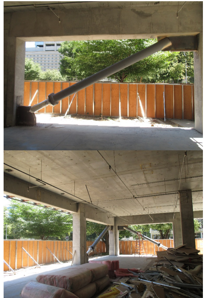
Figure 18. Seismic retrofitting using viscous dampers
