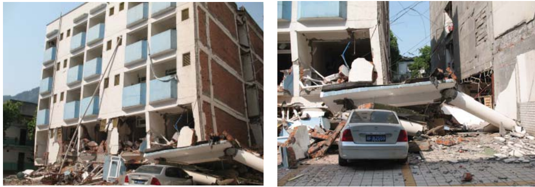
a. Soft story collapse
