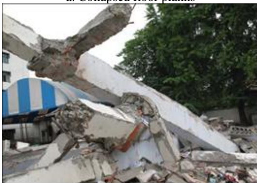
c. Non-ductile CIP-RC beam
