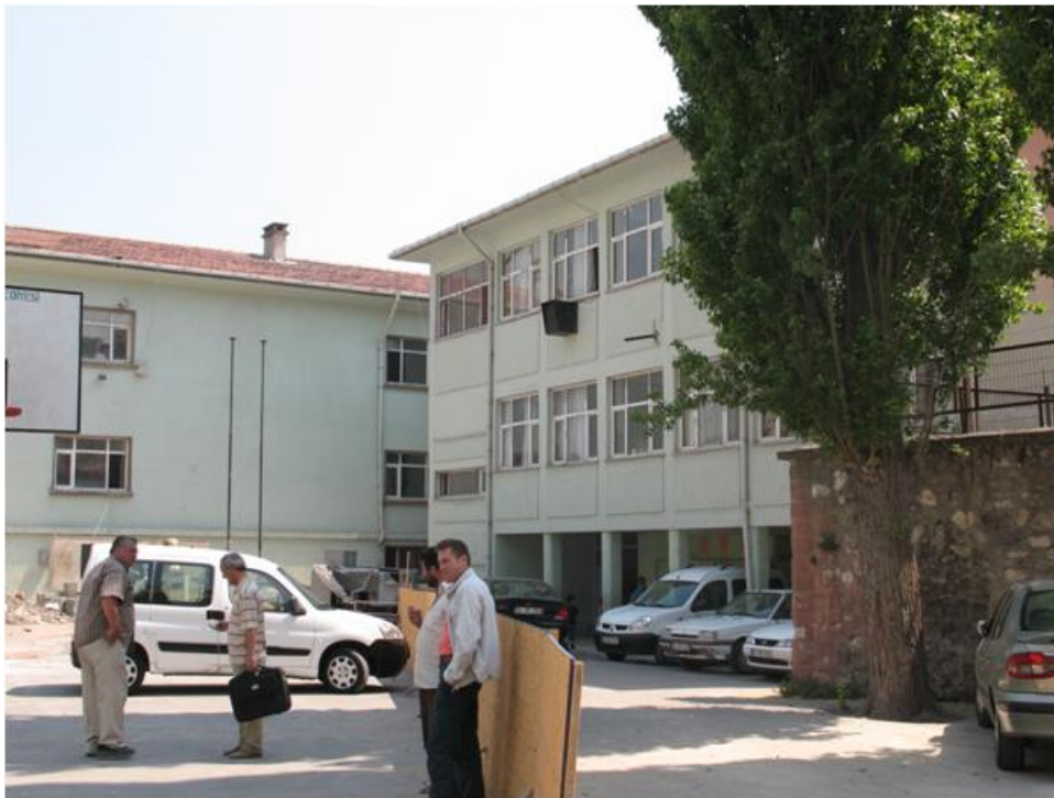
Figure 14. A vulnerable structure
