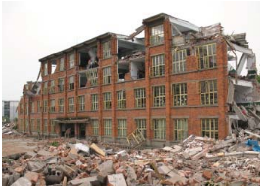
a. Column flexural failure
