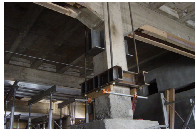
Figure 12: Column with jack frames in place, prior to the construction of the transfer beams
