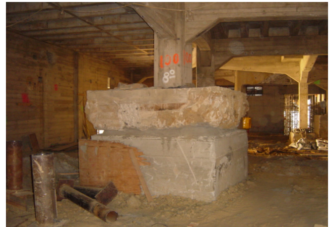
Figure 11: Column footing supported on temporary underpinning
