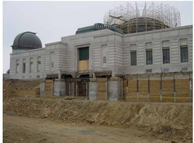
Figure 8: Existing building showing underpinning at entrance
