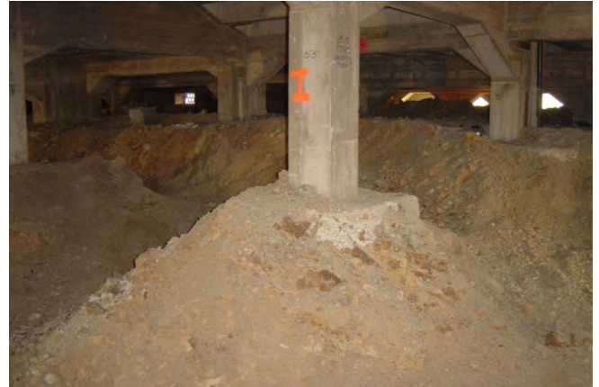
Figure 10: Excavation around existing column footings
